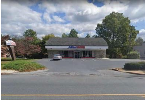
Excessive Existing Curb Cut width
